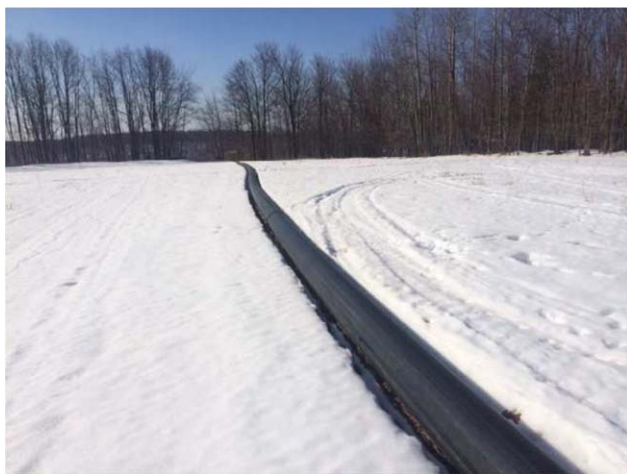
Figure 5. Water transportation through temporary piping.
